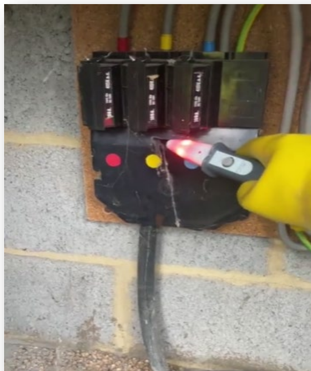
Figure 1 - Contact voltage detector being used to test for a voltage appearing on the outer enclosure of the service head (Image courtesy of Eddie Clemmens, Pegasus Electrical)
